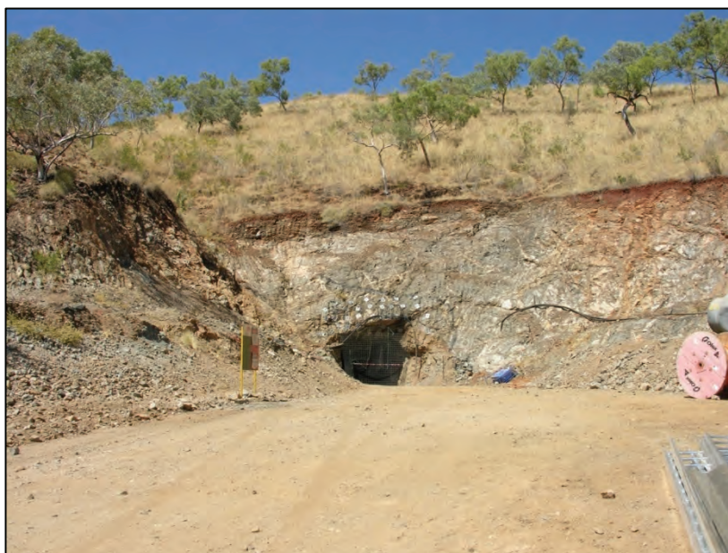
Figure 3: Exploration portal and decline access (source: Company materials)
