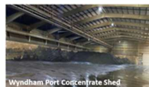
Wyndham Port Concentrate Shed
